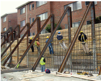
Repairs in full swing at St. Stephen's Court Apartments Wall.
