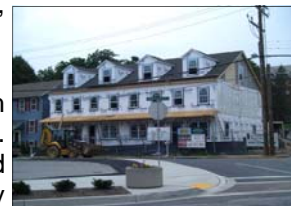
Phases of the on going construction at the Union Crossing project.
